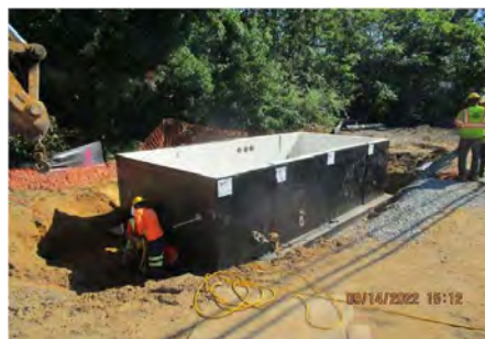
Water Main Construction & Connections
