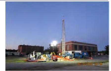
Drilling Potable Well
