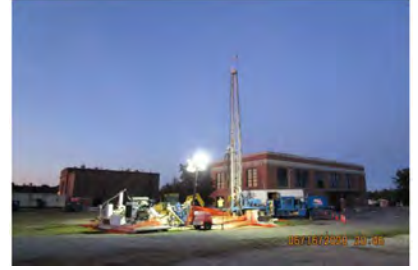
Drilling Potable Well
