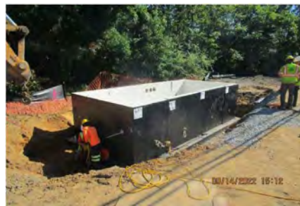
Water Main Construction & Connections
