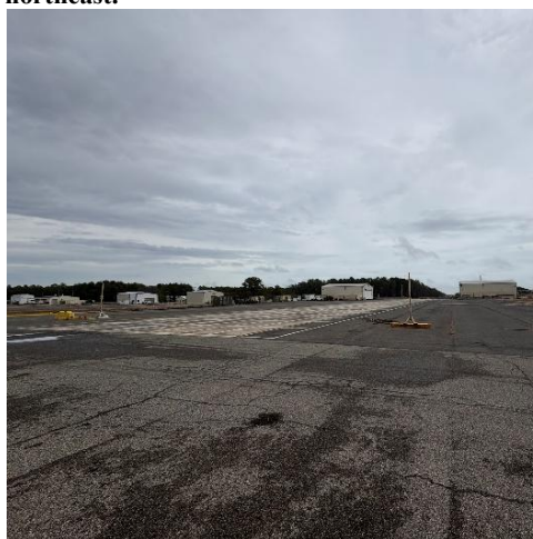
Photo 22: Area K SA004 view facing east.
