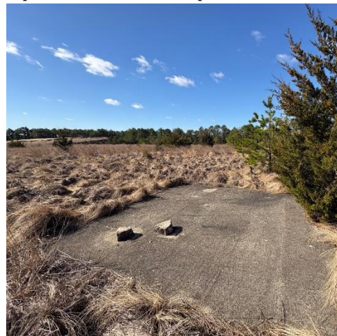
Photo 36: Area D Site LF031 concrete pad near center, looking southwest.
