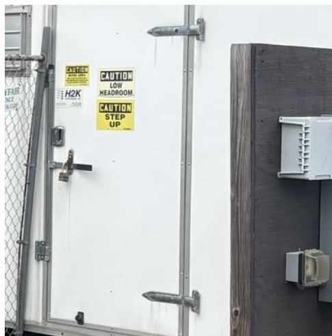
Photo 6: Area A Site LF042 locked door.
