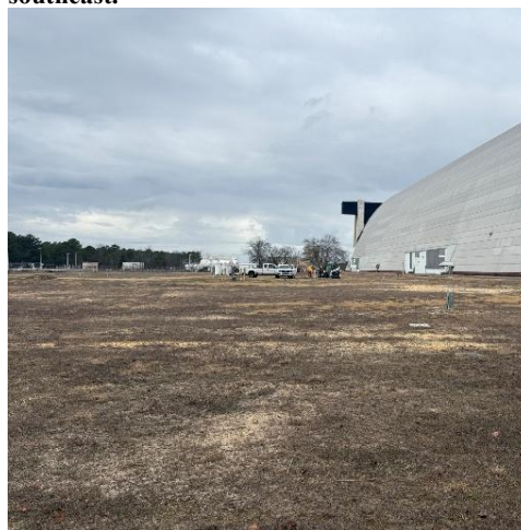
Photo 16: Area C Site TT017 view facing west.
