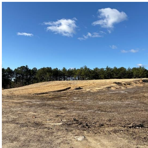
Photo 29: Area D Site LF031 Large soil/ sand stockpile in the southwest corner of landfill.
