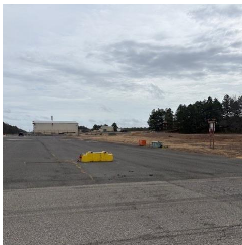
Photo 24: Area K view facing north.
