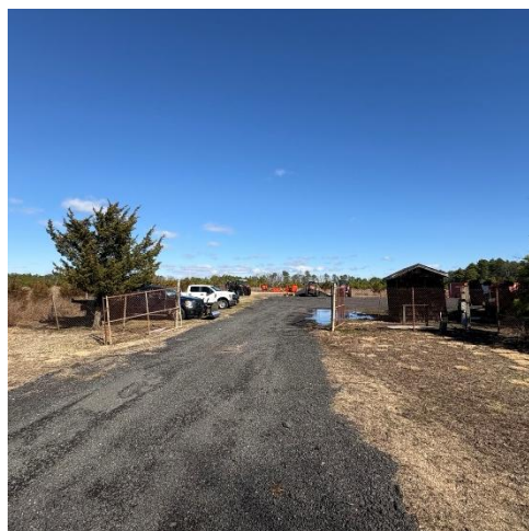
Photo 27: Area D Site LF031 south maintenance entrance.
